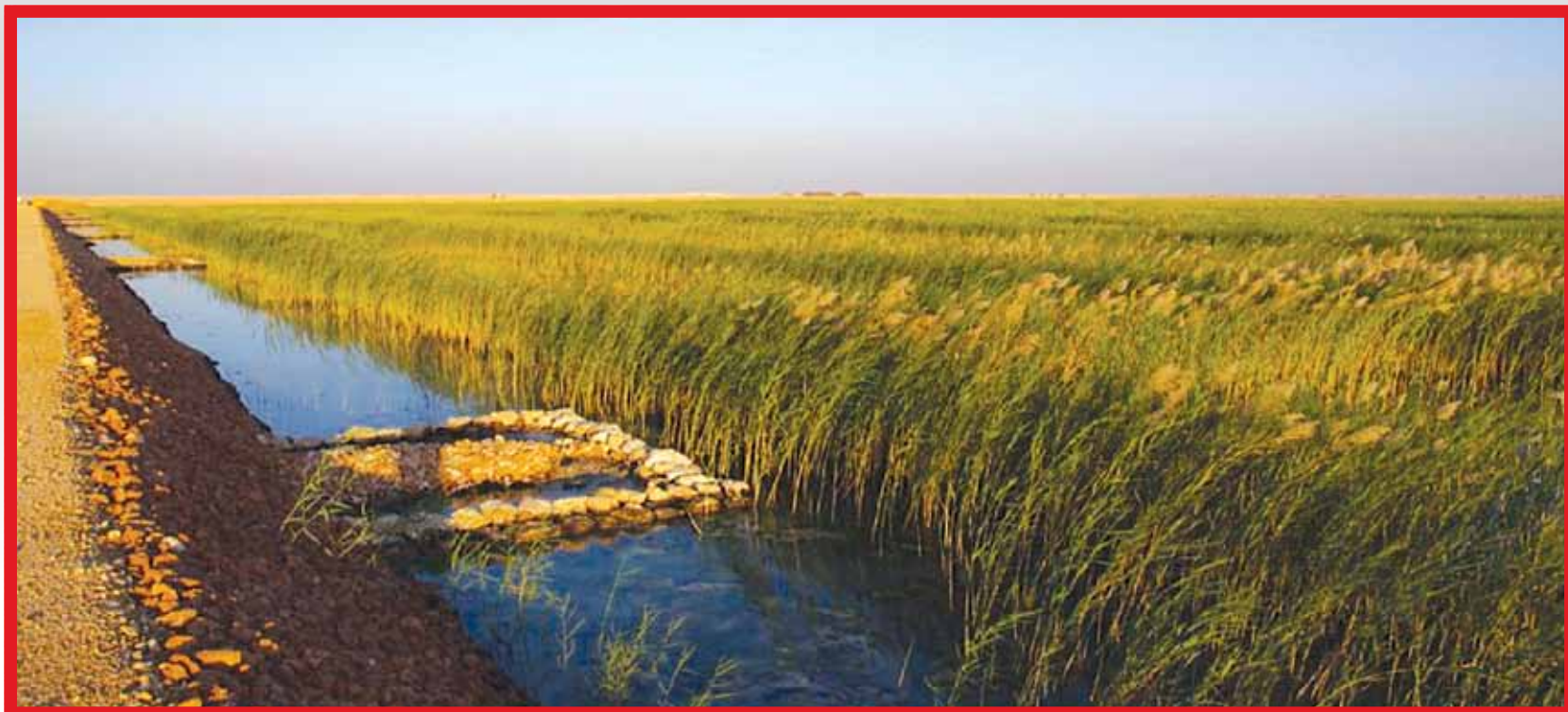
Inlet works on one of the 24 reed bed cells
