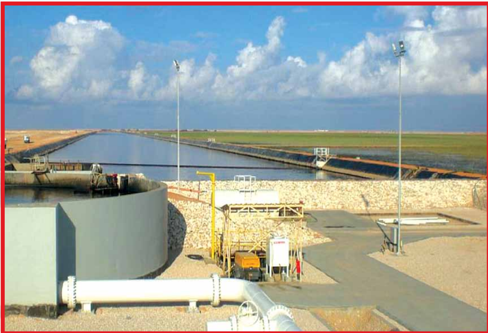
Oil separator, inlet buffer pond and reed beds
